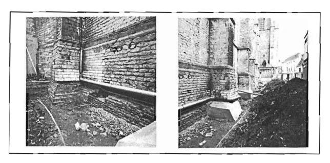
Before deciding on other measures, the upward flow of moisture should be halted. Rising groundwater is often caused by leaking drain pipes or other systems to convey water to the base of a building. A drainage system, installed at ground level, would absorb and drain off water at the base of the facade. In the past, financial factors meant that the base of a building was constructed differently to the rest of the building. In that case, protection is essential.
